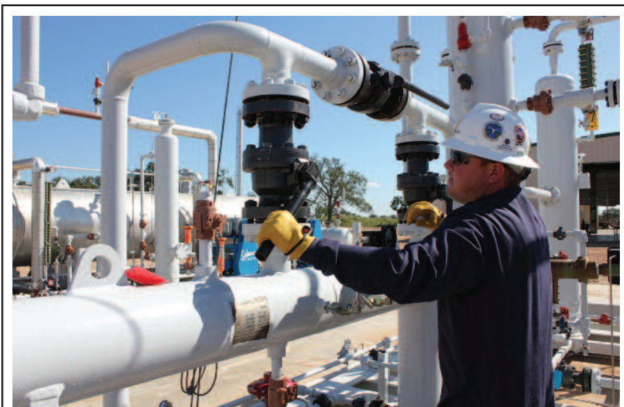
With most of the wells drilled in shale plays yielding multiphase production streams that require some form of treatment, the development of unconventional resource plays has had a significant impact on the natural gas treating industry. And unlike in years past, where natural gas treating companies worked solely at the wellhead, today they also are working hand-in-hand with producers on the front end to develop H 2 S and CO 2 emission strategies for centralized production facilities and associated drilling programs.
